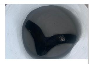
Above: Completed manhole rehabilitation in Clinton, AR, lined with Epoxytec CPP 454 for long-term protection against H<sub>2</sub>S and infiltration.
