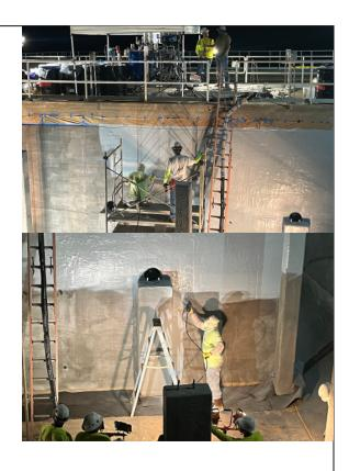
Above: Crews apply Epoxytec Series 457 CPP Sprayliner 61 to basin walls at Bonham WTP while the plural-component equipment operates from above.
