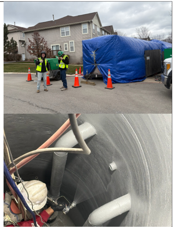
Top Image: Insituform technicians with the enclosed worksite structure that provided critical environmental control during cold weather application, helping maintain optimal temperature for the Series 456 CPP Sprayliner curing process.
