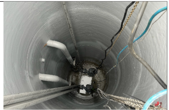
Close-up view of the completed coating application in the wet well, showing the seamless protective barrier.
