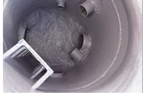
Above: Manhole after concrete restoration.
