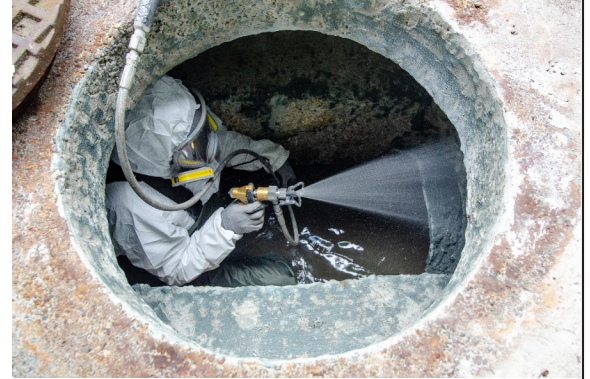
Above: Series 451 CPP Sprayliner MH being sprayed on substrate.
