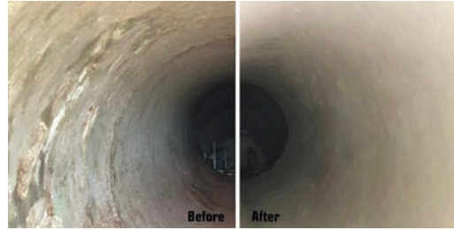
A before-and-after look at the results of lining a pipe with Epoxytec.
