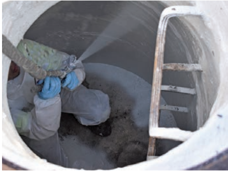
Epoxytec provides a variety of rehabilitative and lining solutions, focusing on applied, immersion rehab and lining products that protect against H 2 S and seal against I&I.
