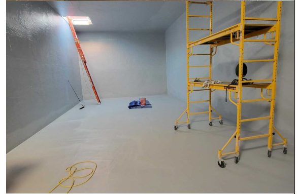
Above: before and after being lined with CPP Sprayliner.
