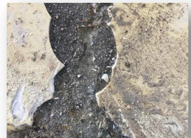
Cracks drilled to relieve water pressure
