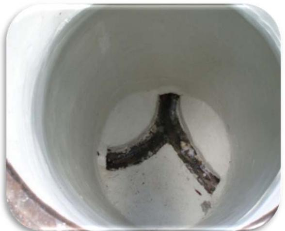
Unless the structure is susceptible to high flow - once applied to the surface, the structure may be returned to service almost immediately – CPP will cure even in wet environments. *Note: if the structure will experience heavy flow, force/pressure, or agitation – let CPP cure for a few hours (4 - 6) before returning the structure to service.*
