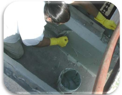
5. **You are now ready to apply CPP™ to the substrate.** You may use a trowel, spatula or blade type device. In some cases, applicators even find using a glove by hand works well.
