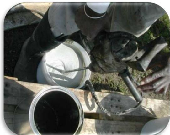
4. **Once you have a good mix, spread the CPP™ out on a mixing board.** Epoxy based products last longer (have an extended pot life) if they are not left in the bucket. The more spread out they are, the longer they last.
